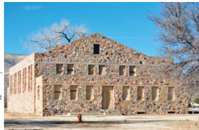
The old gym at Stewart Indian School is among the buildings slated for renovations. The state has approved $4.6 million for renovations and new facilities.
